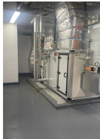
New AHU for emergency waiting area
