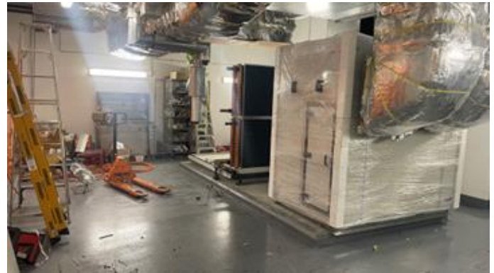
Replacement AHU being rebuilt
