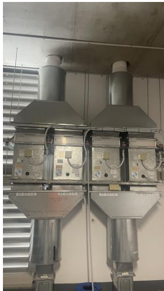
Upgraded duplex exhaust fans for isolation rooms
