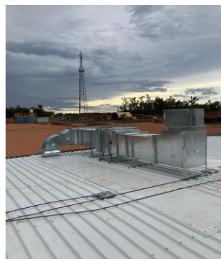
Roof mounted exhaust fan
