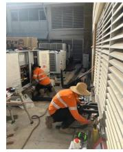
4 new non-essential MSSB's and 1 new essential MSSB were manufactured and installed to replace the existing MSSB's that didn't comply with AS3000 clearance restrictions. New controls for the entire N Block were installed, this was to also include existing mechanical equipment that wasn't replaced as part of the works.
