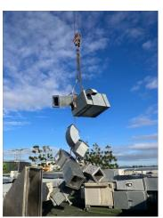
Scope of works was to decommission and remove 13 rooftop package units, existing MSSB and other associated equipment. Mitsubishi Electric VRF systems were installed which entailed 14 condensers to 25 split ducted units and 7 in ceiling cassettes along with 26 fans and 6 roof cowls and 1 new MSSB to provide power to all new mechanical equipment.
