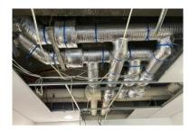
The work, undertaken during the end of year semester break, required stripping of the existing lagging and sheathing, replacement of the thermobreak insulation, and the external metal sheathing replacement to the system.
